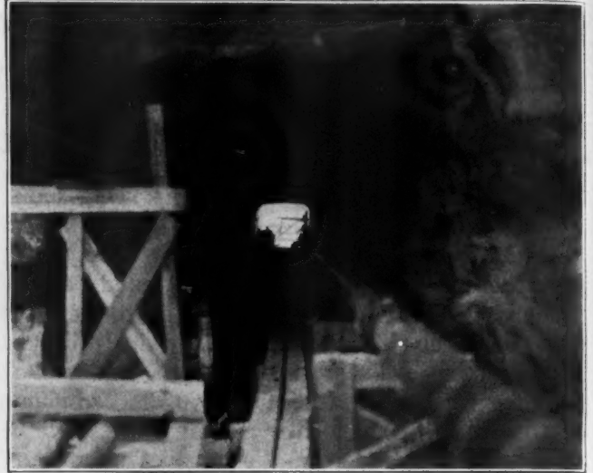
Tunnel Leading Under Street Railway Tracks to Operations on Opposite Side
